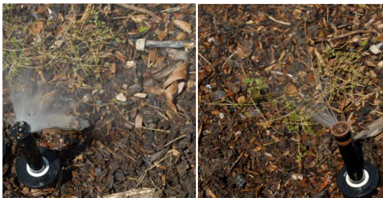
The image at left shows a spray sprinkler with a body that is non-pressure-compensating, resulting in water wasted from misting and overwatering. The image at right shows a pressure-regulating spray sprinkler body that regulates the water pressure to the sprinkler nozzle's optimal pressure.
